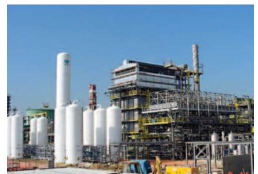
Spain - 60,000 Nm 3 /h Hydrogen
