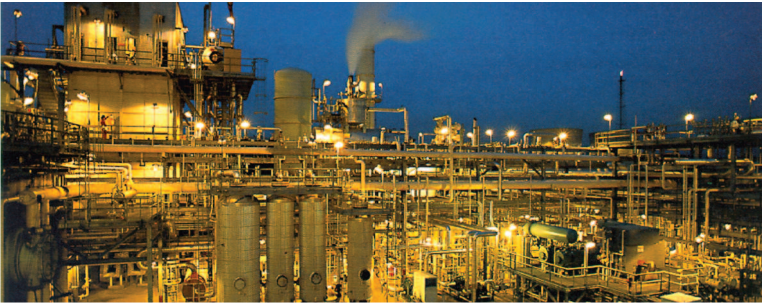
USA - 48,000 Nm 3 /h Hydrogen
